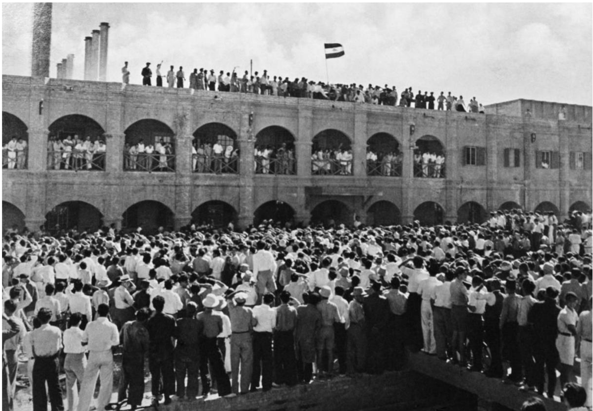
Figure 1. 'Iranian Flag raised above Abadan Refinery, 24 June 1951.' Source: ARC78148, BP.
